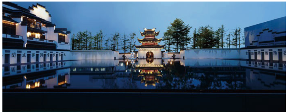
Facade & Landscape Lighting
